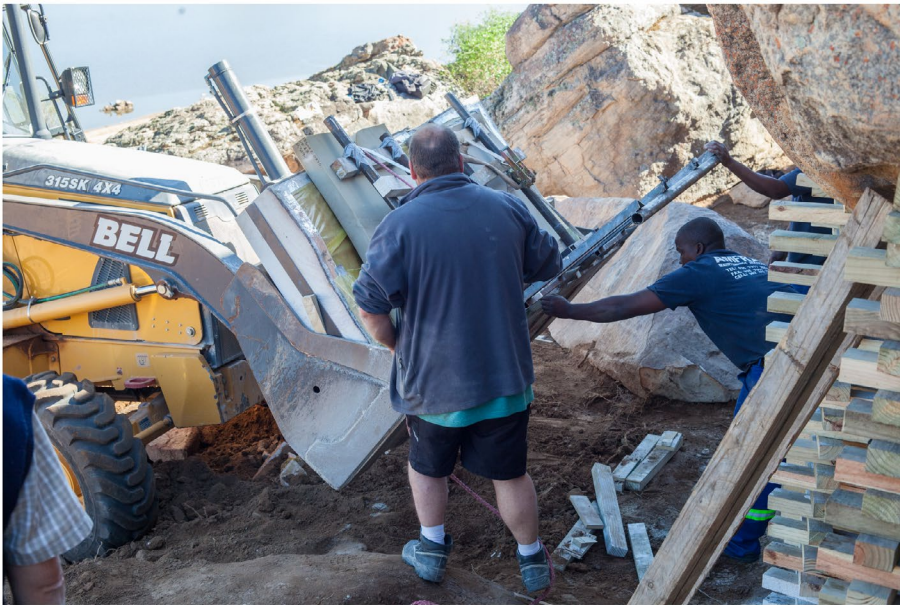
Figure 18. The painted block from Site CDE02, still strapped to its cradle and with a short section of rails, is loaded into the carrier bucket of a TLB.
