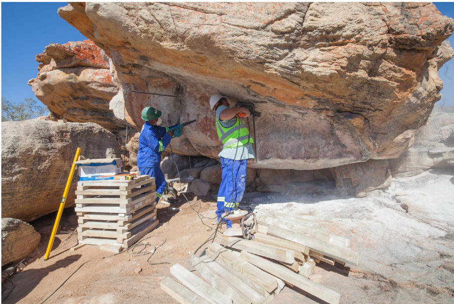
Figure 21. Site CDW10, the second site from which rock art was removed. Guide cuts for the diamond wire saw are being dry cut with the double-bladed rotary cutter. A blower is used while cutting in order to keep dust from settling on the rock art.
