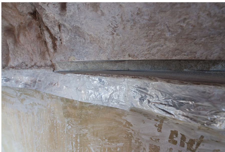
Figure 15. The top cut along the top of the block at Site CDE02 varied in depth between 150 and 350 mm and was made with a double-bladed rotary cutter that was cooled with water.
