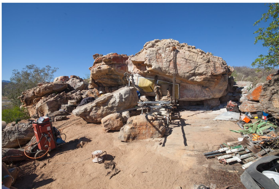
Figure 22. The diamond wire saw set up for cutting at Site CDW10. The wire saw is controlled from the console at left.
