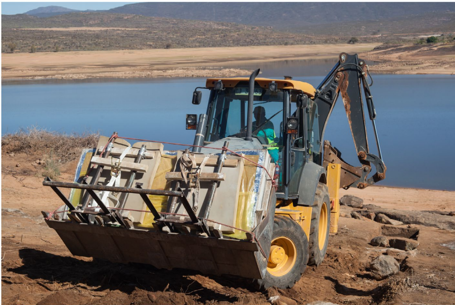
Figure 19. The block of rock from Site CDE02 on a TLB loaned by Department of Water and Sanitation on its way to temporary storage in the nearby town of Clanwilliam.
