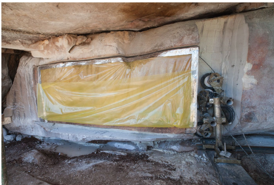
Figure 14. The rock art at Site CDE02 was waterproofed with plastic sheeting, aluminium tape and silicone. The pulleys at right are part of the diamond wire saw setup.
