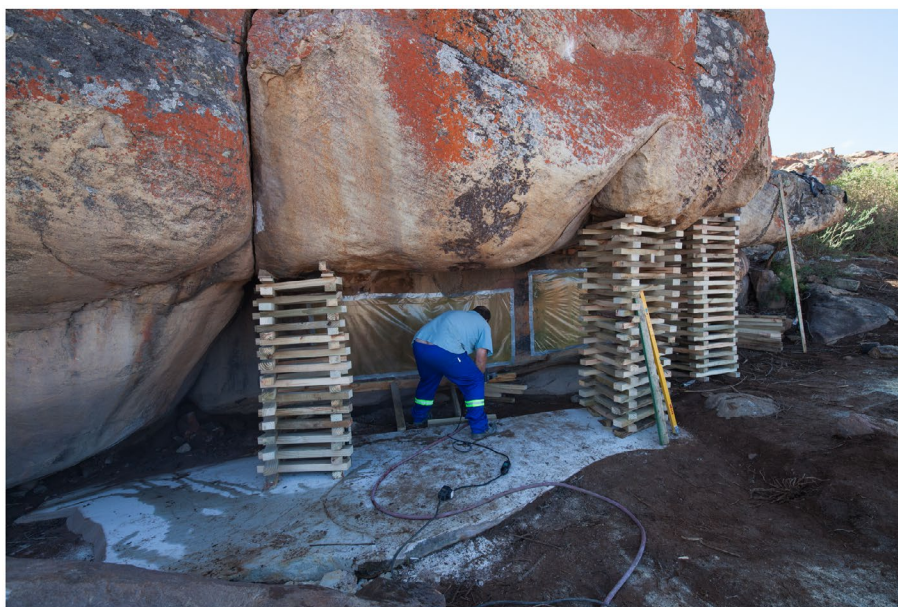
Figure 10. The overhang at Site CDE02 was reinforced with wooden packs to support the rock mass above the paintings.
