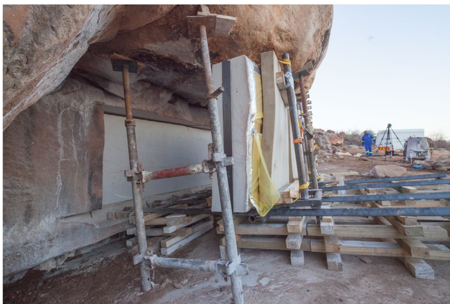
Figure 17. The block at Site CDE02 has been cut free and has been wheeled from underneath the overhang on a cradle on rails.
