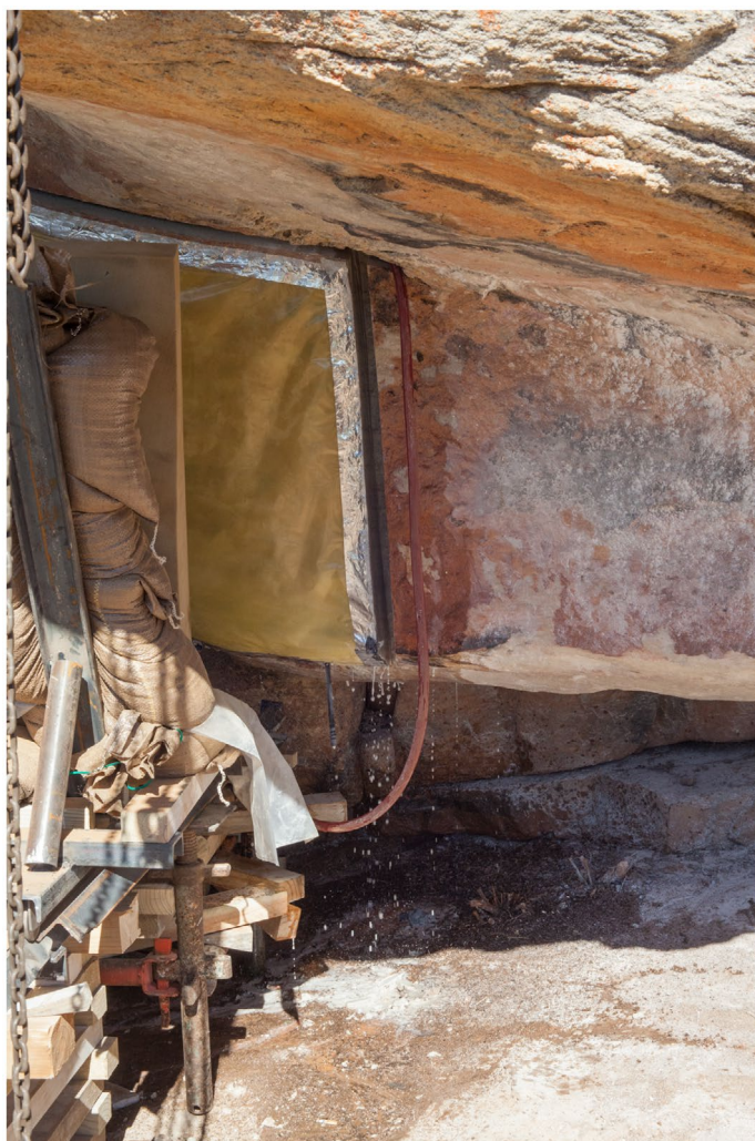
Figure 23. Water-cooling the diamond saw at Site CDW10. The red hose is feeding water into the cut that the diamond saw is making. A thin slurry of water and dust drains to the ground.
